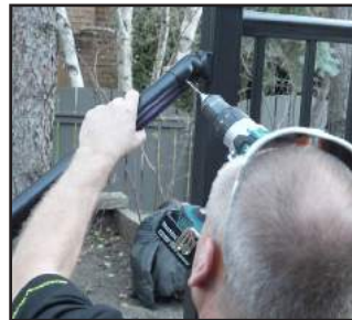
Pre-drill and secure top rail into top swivel bracket using URCS50 screws (sold separately).
