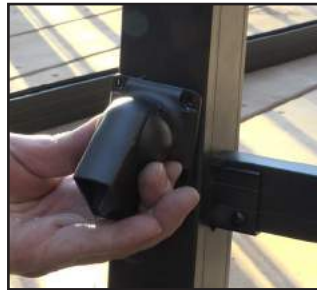
Proper position of bracket is with bottom rail "arc" at top.
