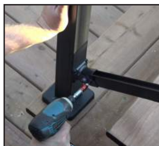
Use URCS50 screws (sold separately) to fasten swivel bracket to bottom rail.
