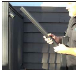
Install top rail into swivel bracket sleeves
