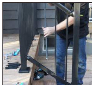
Install pickets and spacers as described in previous "installing pickets" paragraph to complete the stair rail section.
