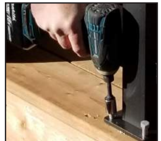
Tighten post bolts/ lags
