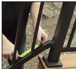
! Spacing between pickets should not exceed 4"
