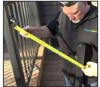
Measure for rail length and cut rails.
