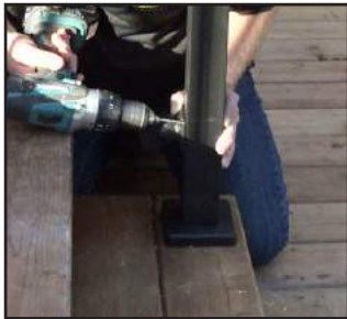
Pre-drill and use URCS50 screws to attach bracket flange at this height.
