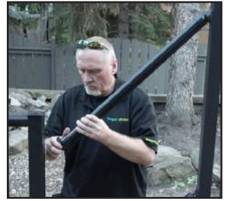
Slide top swivel bracket onto top rail.
