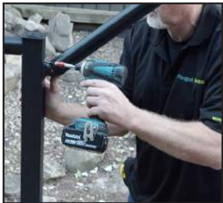
Secure top swivel bracket into post using URCS50 screws (sold separately).
