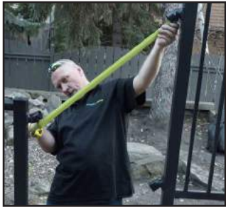
Measure distance between inside of swivel brackets and cut top and bottom rail to fit.
