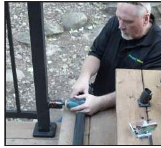
Remove ONE SIDE ONLY of bottom swivel brackets.
