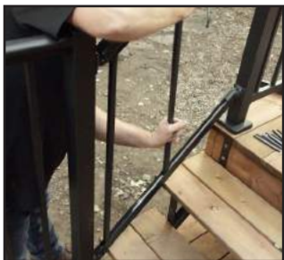
Install pickets and spacers as described in previous "installing pickets" paragraph to complete the stair rail section.
