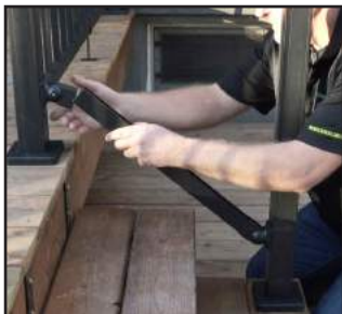
Loosen bolts/lags holding bottom stair post, allowing room for top and bottom rails to slide into bracket sleeves.
