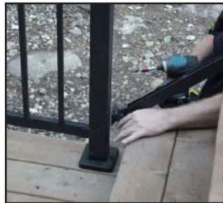
Secure bottom swivel bracket into post using URCS50 screws (sold separately).
